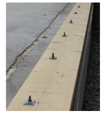
Sill fixed in base with sill nail.
