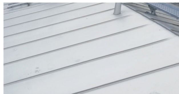
Roof tin sheets on the existing roof.
