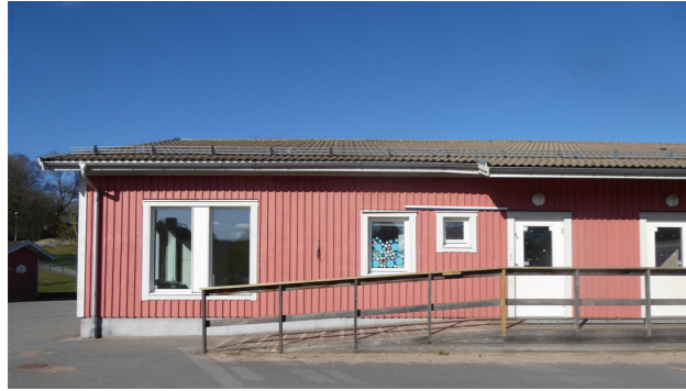
Facade of Biskopsgatan 8.
